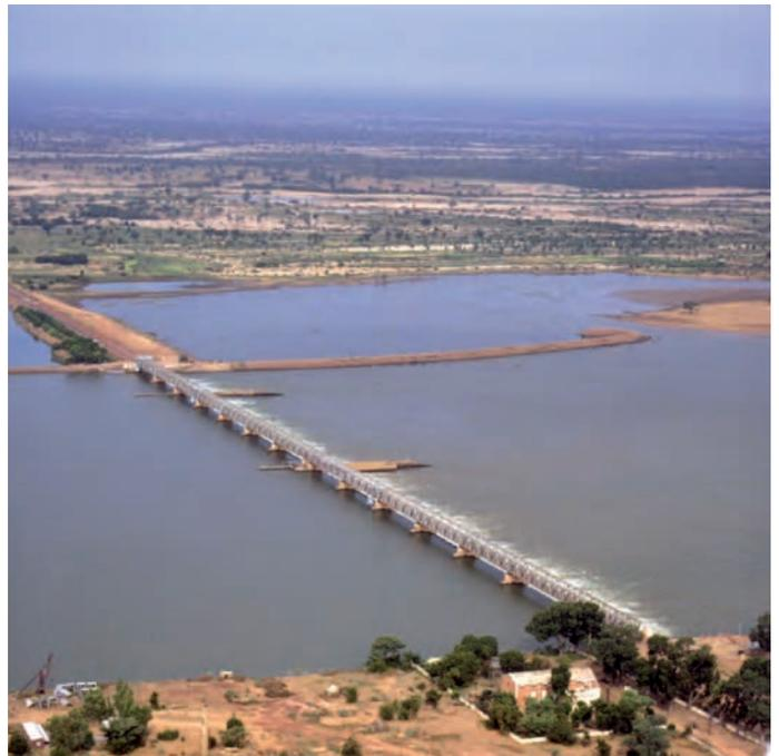
Markala dam on the Niger River near Segou, November 1999. This dam has been operational since 1947 to irrigate the rice fields managed by Office du Niger in the Delta mort, an ancient branch of the Niger.
