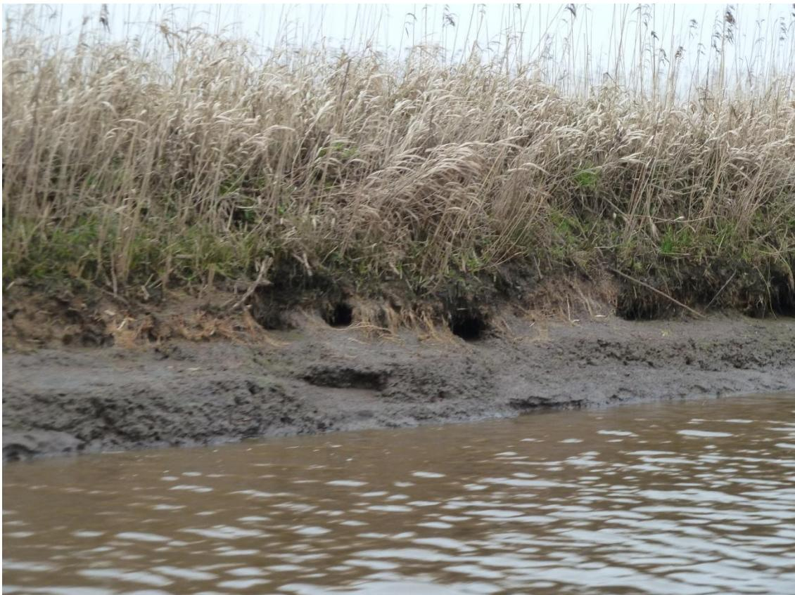
Photo 6.5 Outer slope of the levee along the Veendiep canal, during lowering of the water level to facilitate inspection. Several burrow entrances can be seen. March 2012. Photo Marc Rothengatter.
