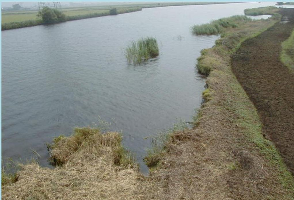
*Photo 6.2: Levee at risk due to erosion after damage by burrowing by Muskrat (courtesy LCCM)*
